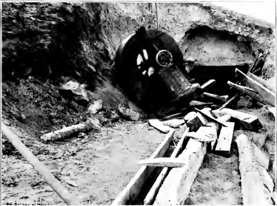
Diamond Vale Colliery—showing Fun as thrown by Explosion.
